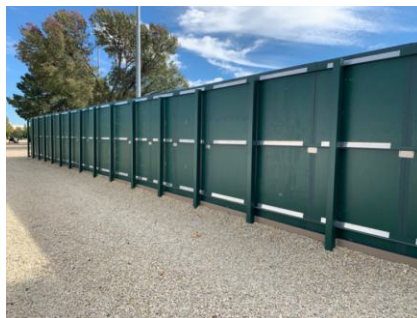
Finished backside view
